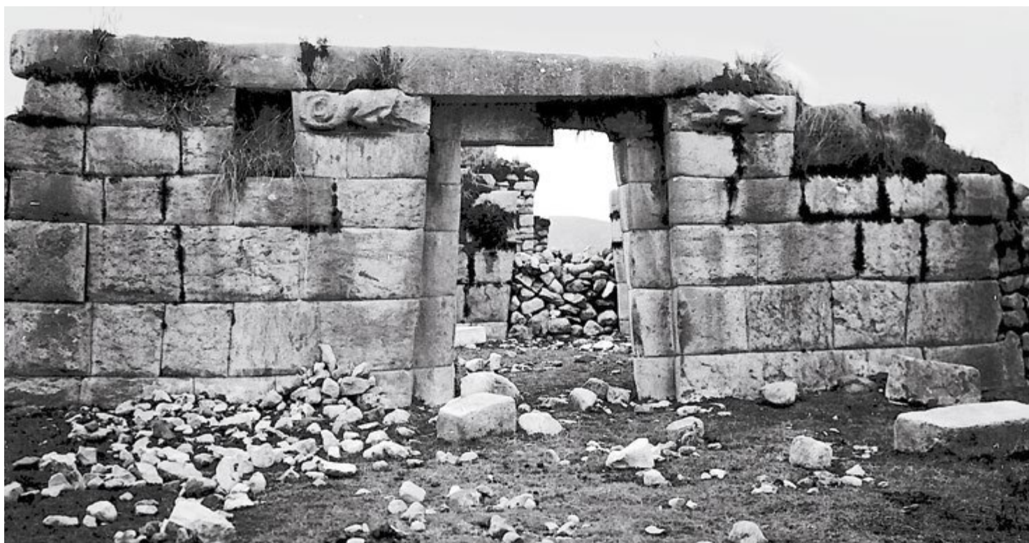
Figure 7 Portal, Huánuco Pampa in 1923. Note that a piece of the lintel has been knocked out. Photograph CSA4644 by John Todd Zimmer courtesy of the Field Museum of Natural History.
